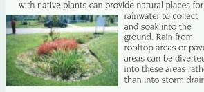
rainwater to collect and soak into the ground. Rain from rooftop areas or paved areas can be diverted into these areas rather than into storm drains.
