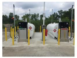
The existing underground gas and diesel tanks at the Public Works building are coming to the end of their useful lives. The Department of Public Works will replace both tanks to properly store the fuel. Both tanks are aging, and over time can become less safe for fuel storage, increasing the chances for seepage and environmental contamination. Replacing the underground tanks with new above-ground tanks will ensure that the contents are stored safely without the likelihood of a subterranean leak.
